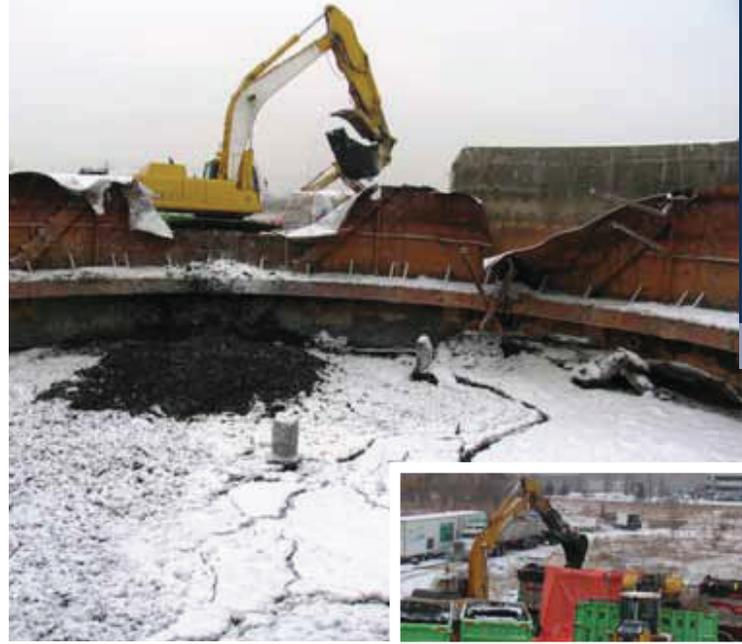
Tri-Phase Environmental Inc. (TPEI) was contracted by the Ministry of Environment (MOE) in December 2010 to remediate a sewage treatment digester tank, with a capacity of three million litres and containing more than 1,500 cubic metres of sludge. The sludge contained high levels of heavy metals, but more importantly, polychlorinated biphenyl (PCB) levels in excess of 50 parts per million (ppm). These high levels classified the sludge as PCB waste as defined by the ministry's regulations.
